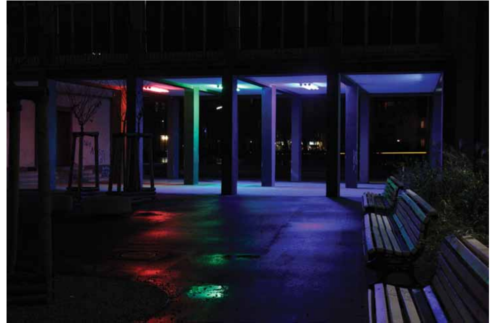
Above, colored lights illuminate the passageway beneath the Haus der Jugend building, promoting a greater sensation of safety. On the left, the plan of Nauener Platz indicates the position of the lighting equipment
